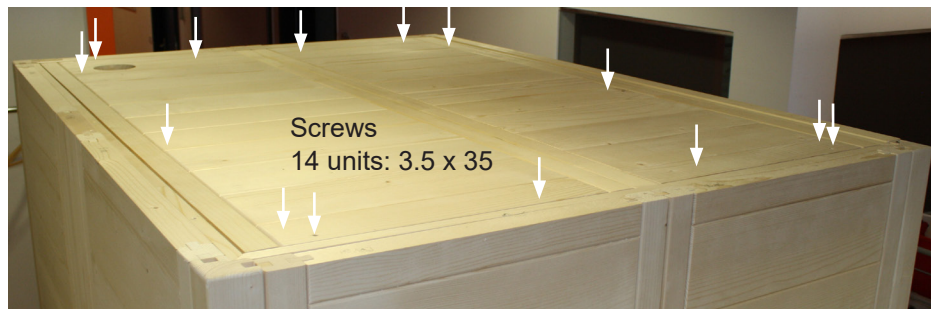
Fig. 18: Attaching the roof element
