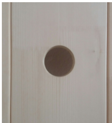
Fig. 38: Installing the control panel
