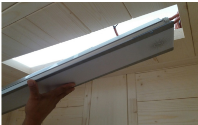
Fig. 44: Installing the colour light
