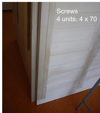
Fig. 46: Installation of the spacer strips of the rear wall
