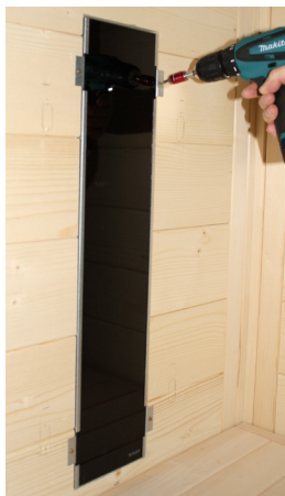
Fig. 36: Install the rear radiator (infrared radiator ECO 350)
