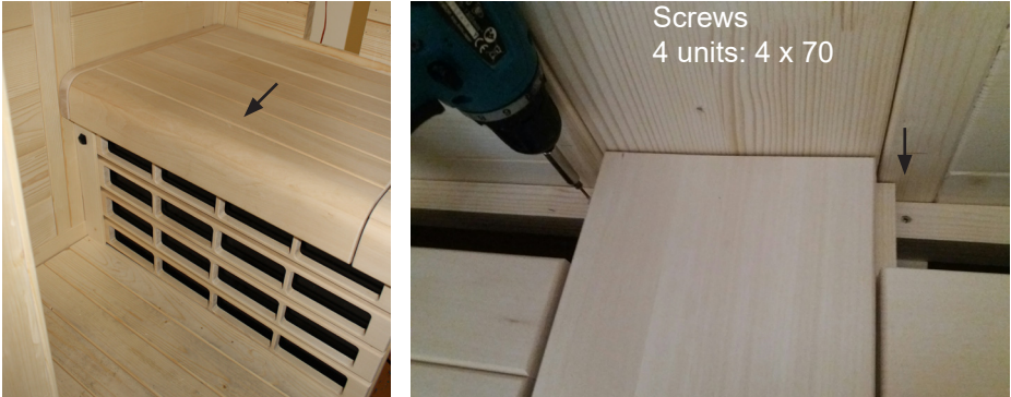
Fig. 45: Attaching the bench
