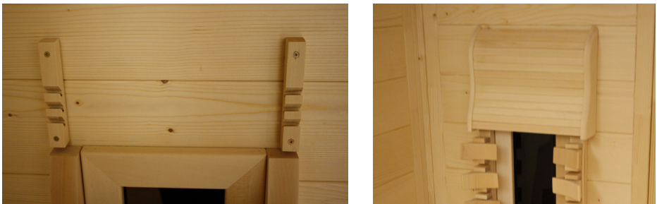
Fig. 47: Installation of the headrests
