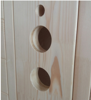
Fig. 43: Installing the control panel
