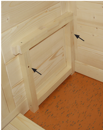
Fig. 30: Installation of the bench cushion
