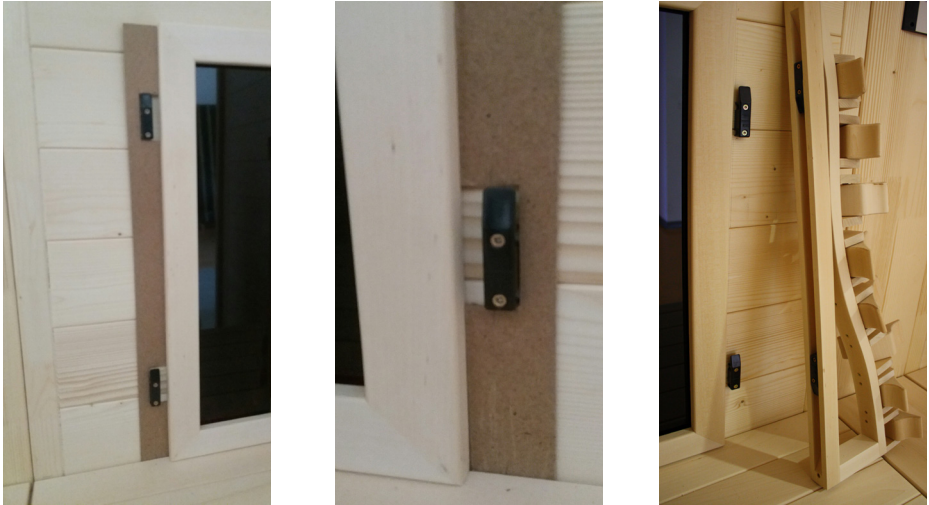
Fig. 48: Installing the backrests of the bench
