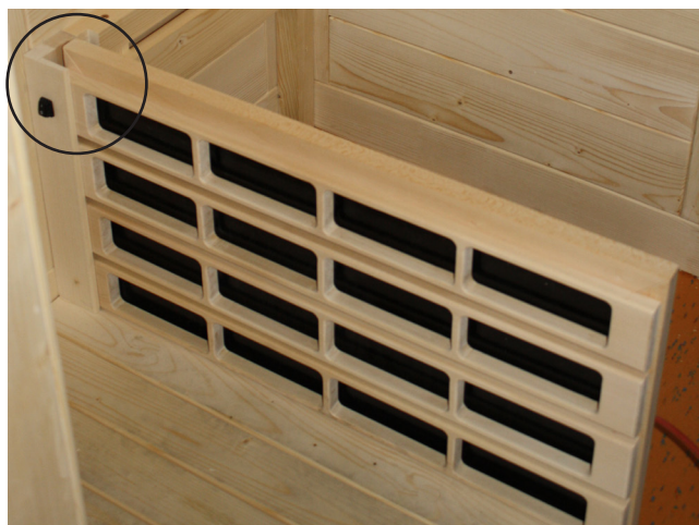
Fig. 32: Installation of the IR thermal plate VitaMy 164
