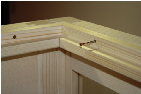
Fig. 14: Roof support slats installation
